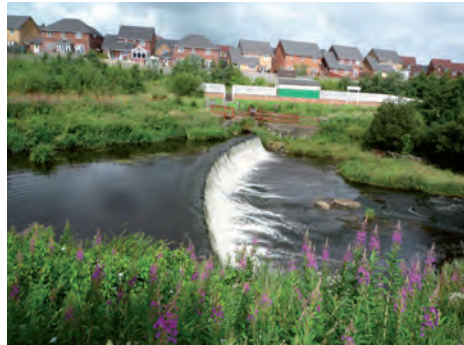
Kirkton Weir, River Almond, Scotland Main constraint: Almond Valley Heritage Centre use leat channel and turbine to produce electricity Option recommended: Formal fish pass
