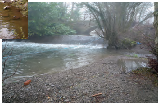
Boulitbrooke Weir, River Lugg, Herefordshire Main constraint: Bridge is a heritage structure. Option recommended: Fish pass
