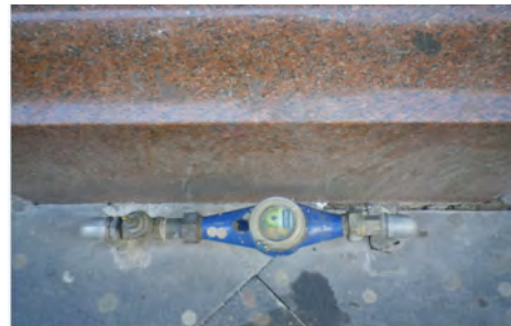
Water meter outside a shop on the high street in Porto Alegre
